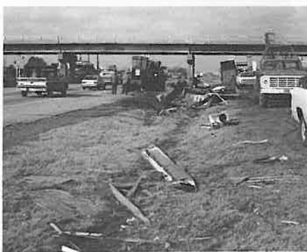
Tornado damage, cleanup in West Memphis
