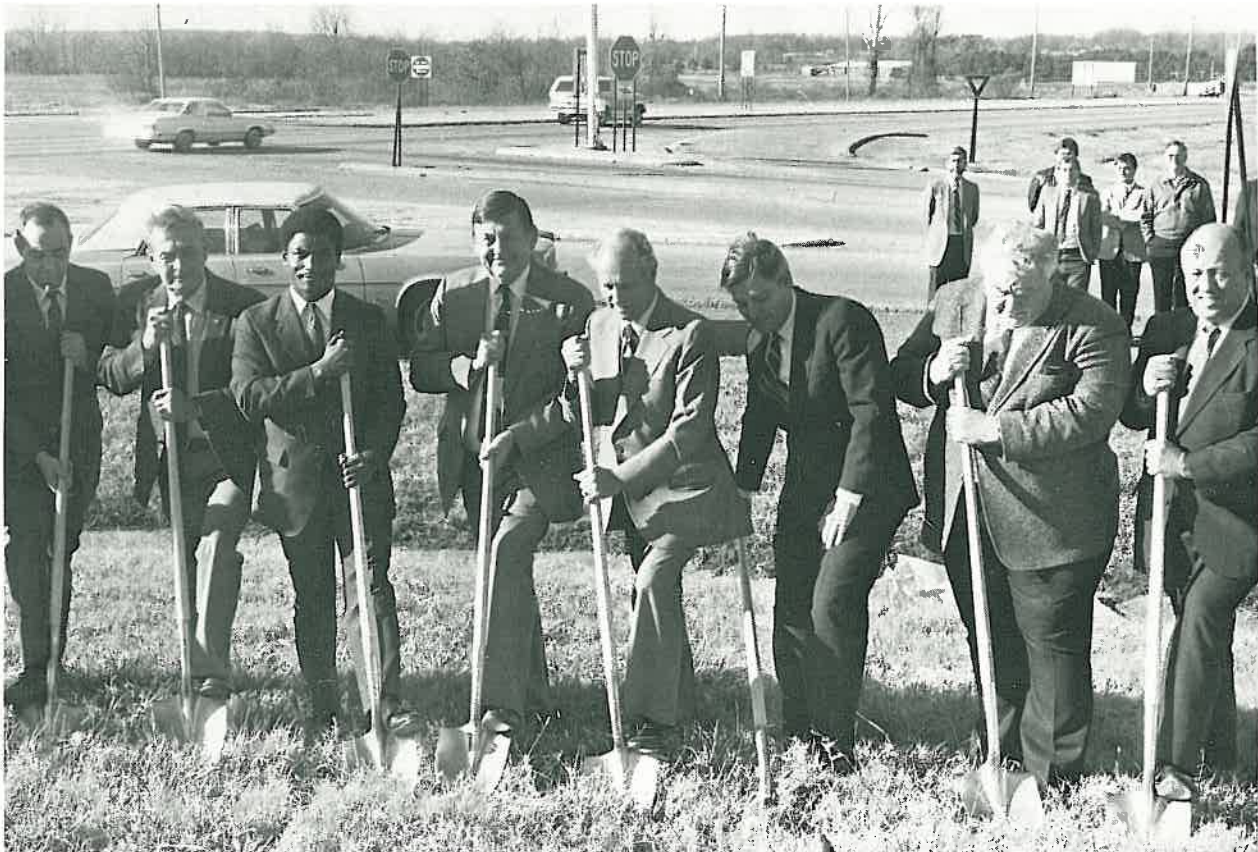
Turning the first shovel of dirt for a new overpass on the Jonesboro Bypass are, left to right, Highway Commissioner Ron Harrod; State Representative Bobby Wood of Jonesboro; Highway Commissioner Rodney Slater; Jonesboro Mayor Hubert Brodell; California Congressman Glenn Anderson; Arkansas Congressman Bill Alexander; Craighead County Judge Roy Bearden; and Highway Commissioner Bill Clark.
